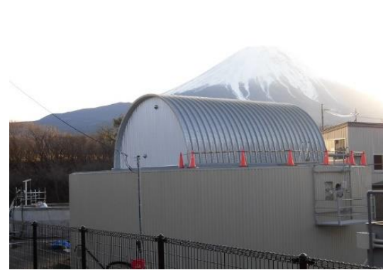
Fermentation tank building
