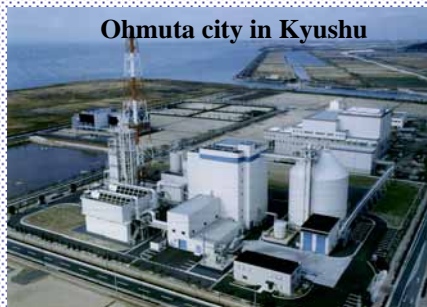
RDF production & combustion - power generation plant
